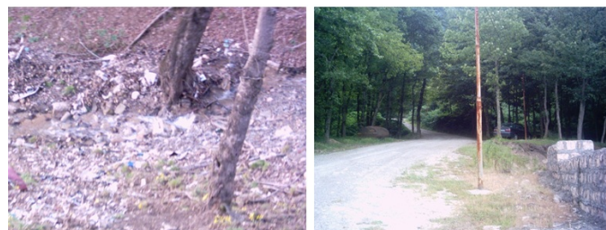
Fig. 3: Access road to the site and the high seepage flow of 10-20 liters per second observed.
