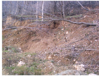
Fig. 2: Scarp of Flourd landslide with tilted trees
